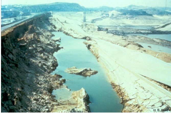
Figure 2. Upstream face of the dam after drawing down the reservoir.
