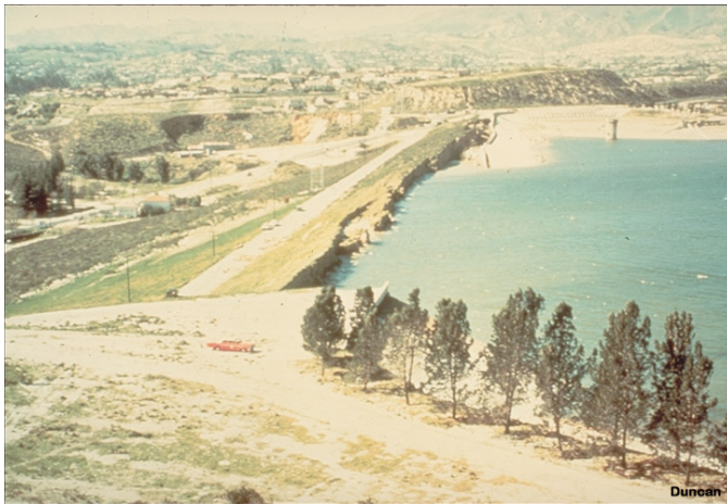
Figure 3. General view of the slide head scarp.
