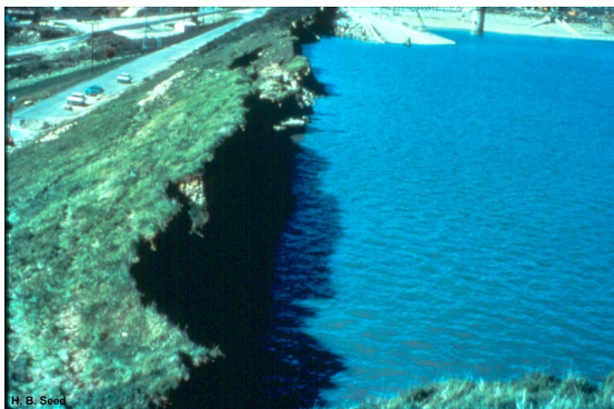
Figure 4. Close-up view of the slide head scarp.
