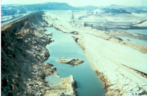
Figure 2. Upstream face of the dam after the drawing down the reservoir.
