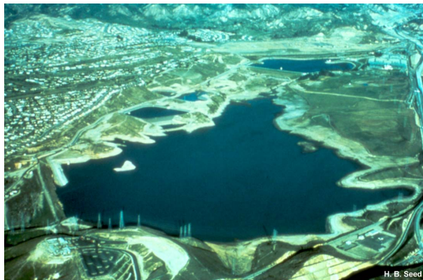
Figure 1. The San Fernando dams and reservoirs.
