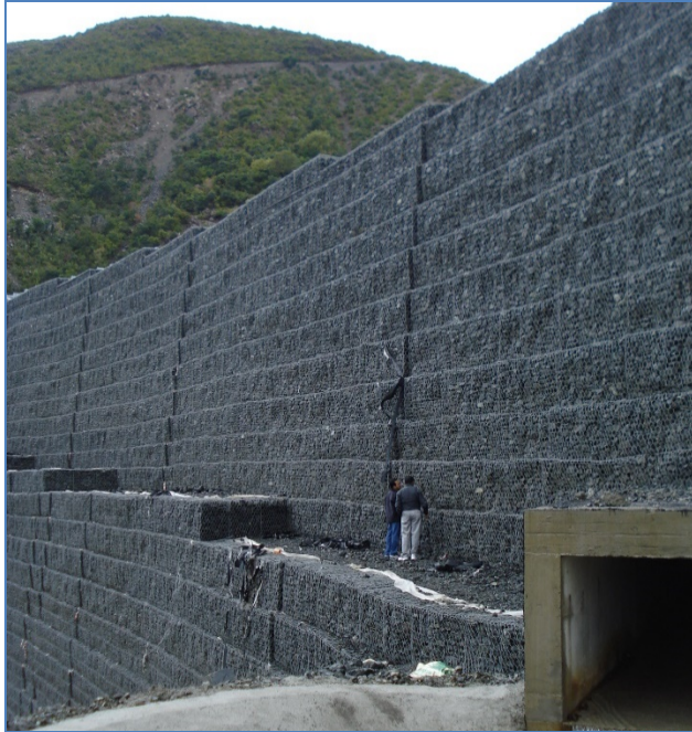
Figure 2. Detailed view of the Maccaferri Terramesh rock wall.
