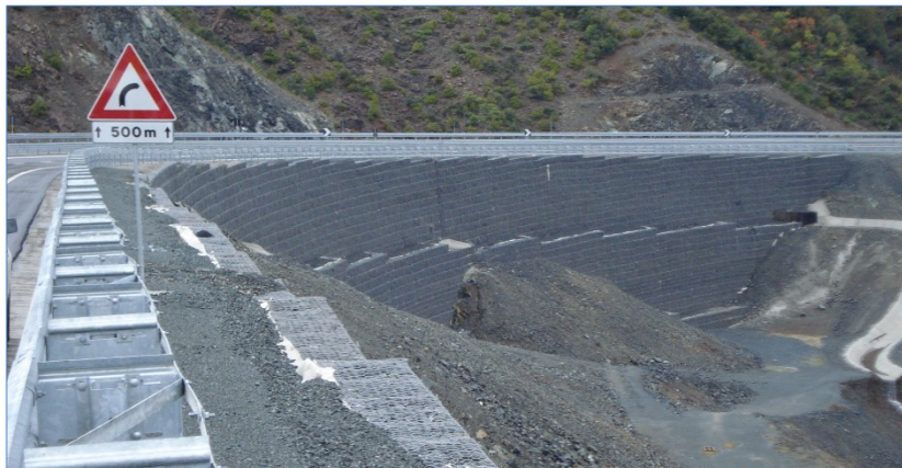
Figure 1. View MSE Wall and roadway.
